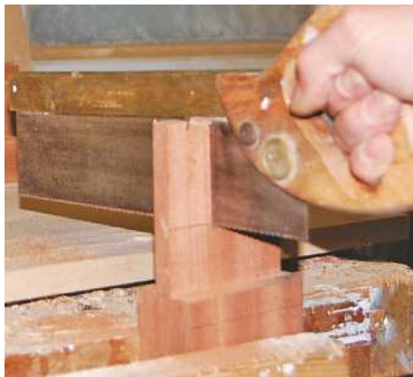
▲ Pic.12 Jason used the waste from the haunches for the wedges on the through-tenons
